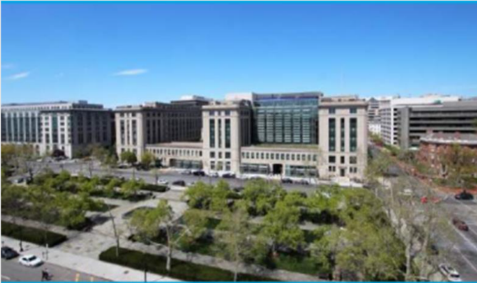
Prototypes were tested at the General Services Administration (GSA) Headquarters in Washington D.C. (Photo from GSA)
